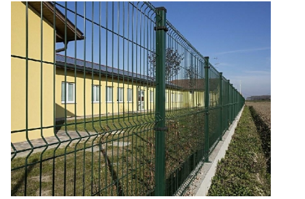
Mesh Weld Fence Example
